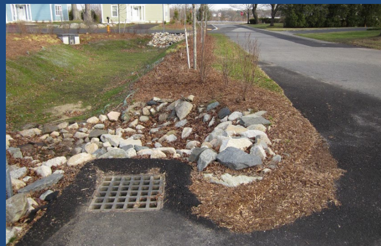
Figure 2.2.3 - Deep-Sump Catch Basin Inlet Structure; Barrington, RI
