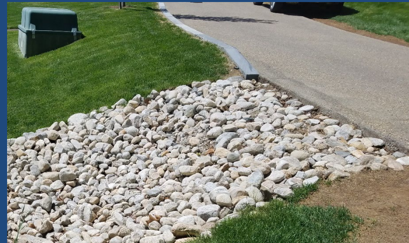
Figure 2.2.4 – Curb Cut with Inlet Protection; Providence College
