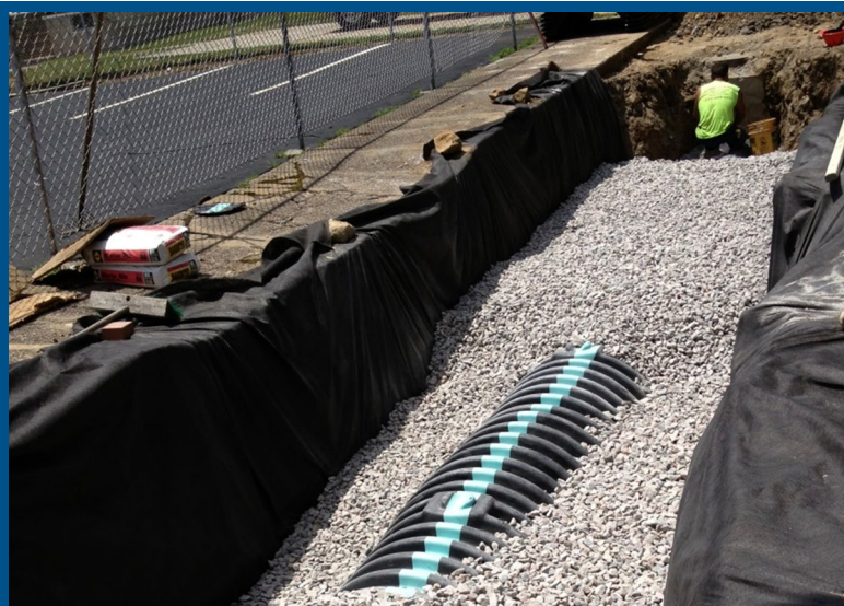
Figure 2.3.3.5 – Installation of an Infiltration Gutter with Subsurface Chambers; West Warwick, RI
