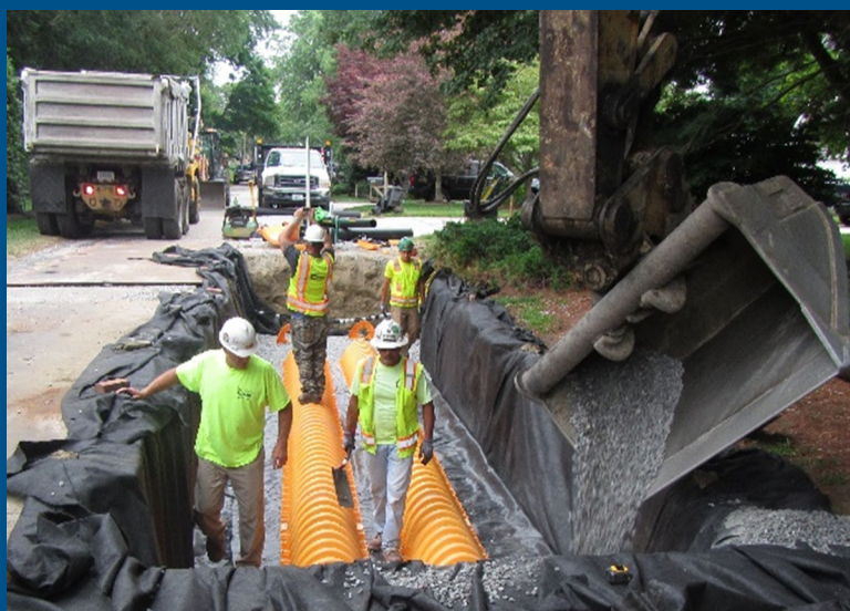
Figure 2.3.3.2 – Installation of an Underground Infiltration System; Narragansett, RI
