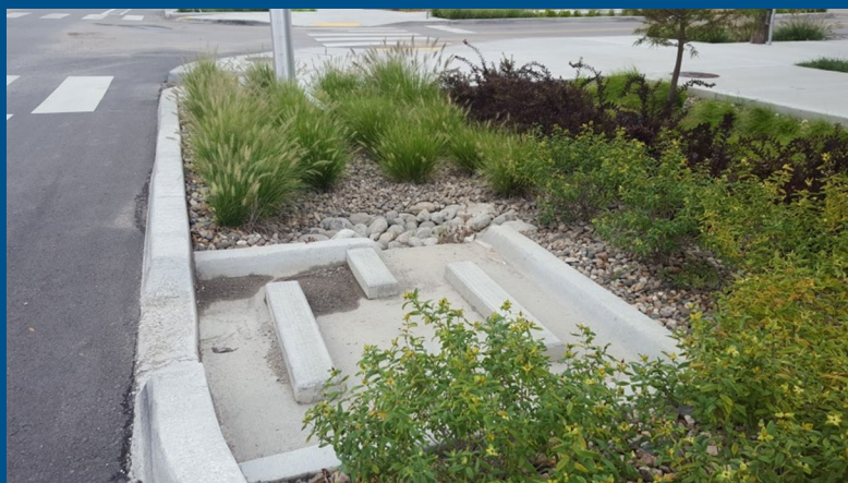
Figure 2.1.2 – Sediment Forebay with Concrete Berms
