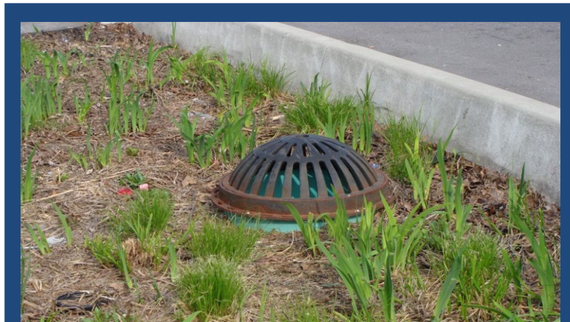
Figure 2.2.6 - Typical Dome Grate Overflow/Outlet Structure; NACTO
