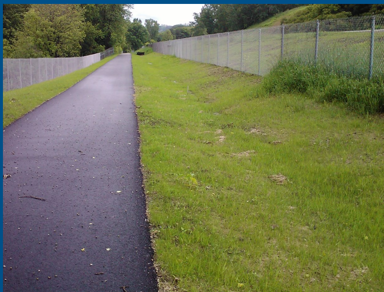
Figure 2.1.3 – Vegetated Swale
